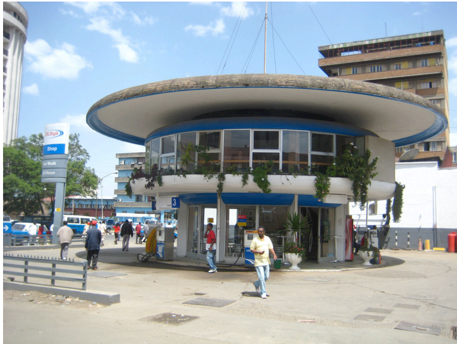
Addis Gojo Style Gas station, Churchill road, 2009
