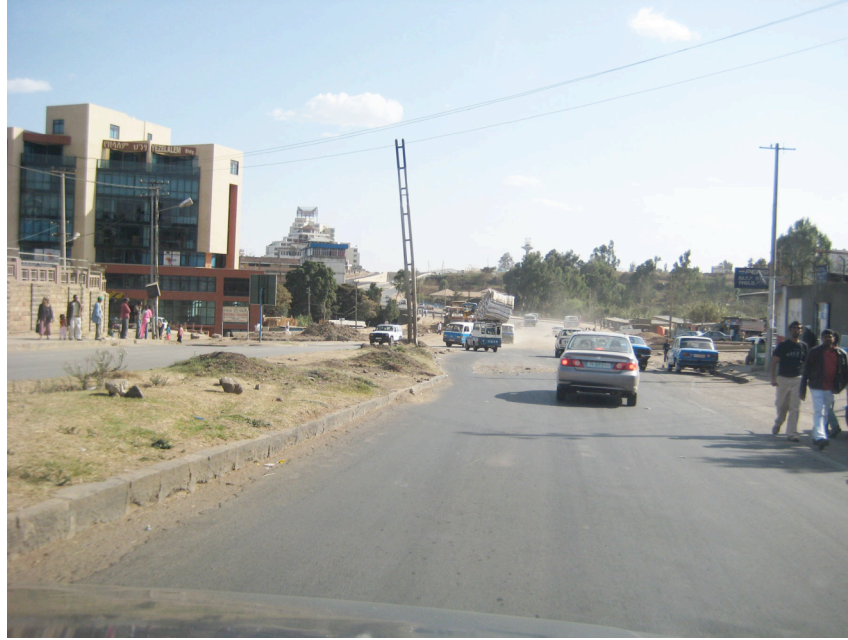
Addis Ring Road Construction, 2009
