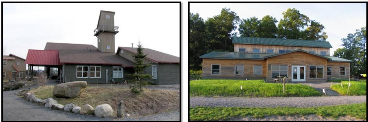
Figure 4.16 Ecovillage at Ithaca's common houses. (l) FROG's (r) SONG's 99
