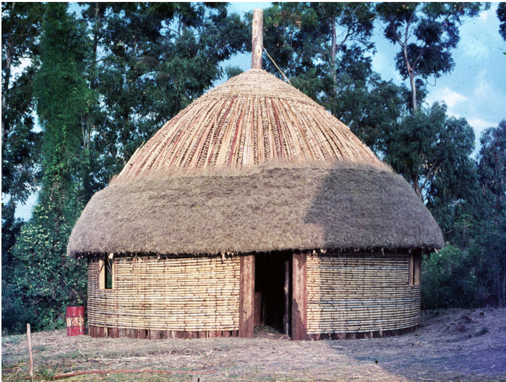
Progress in thatching the roof.
