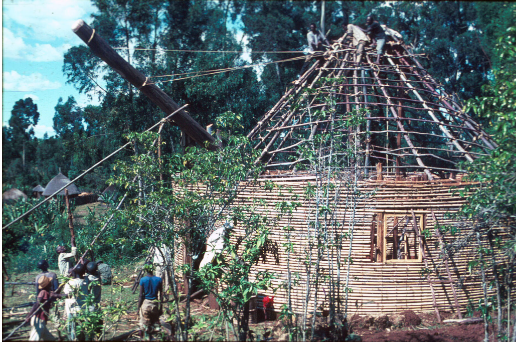
Workers atop the scaffolding pulling the centerpost to vertical position.
