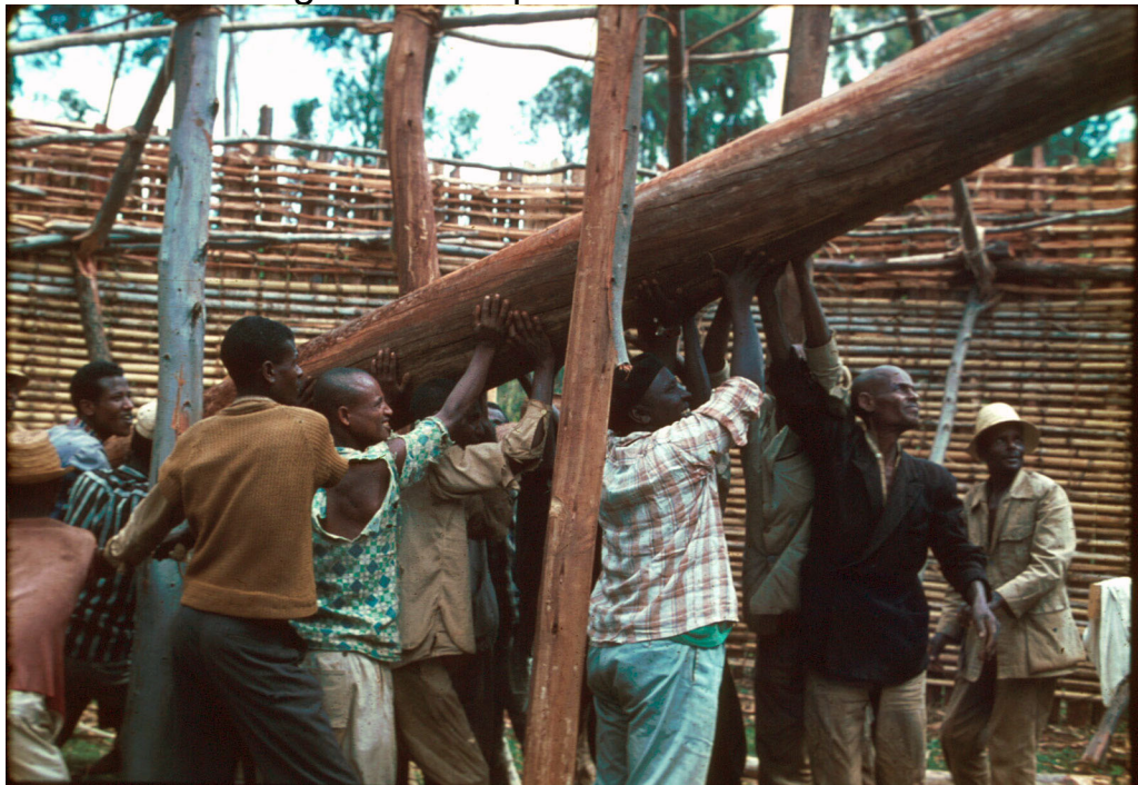
Raising the centerpost with wooden levers.
