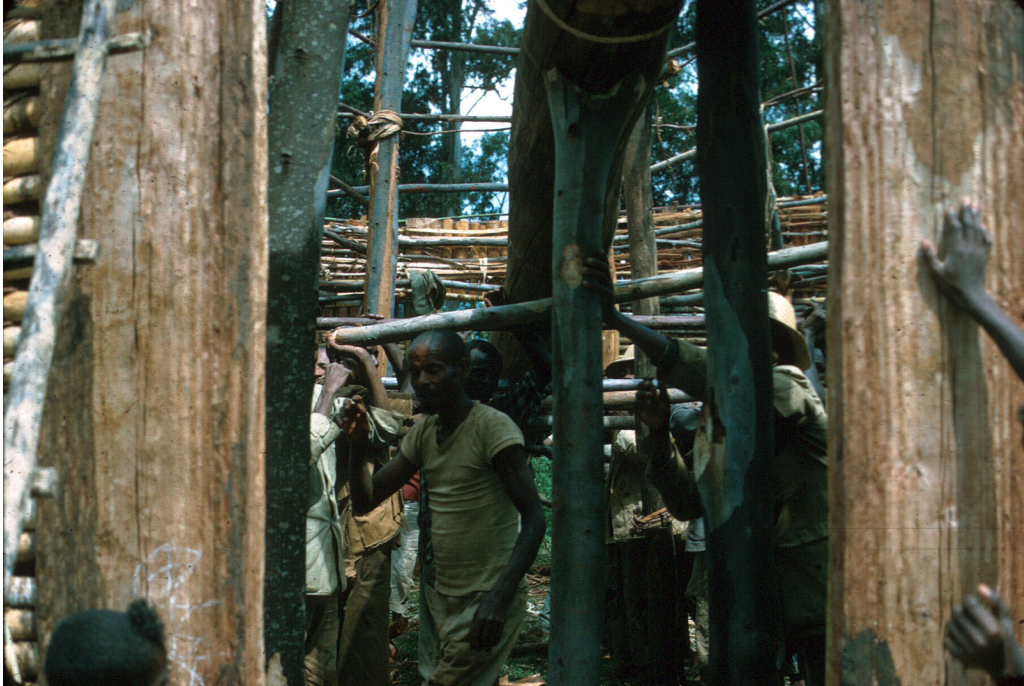
Raising the centerpost with wooden levers.
