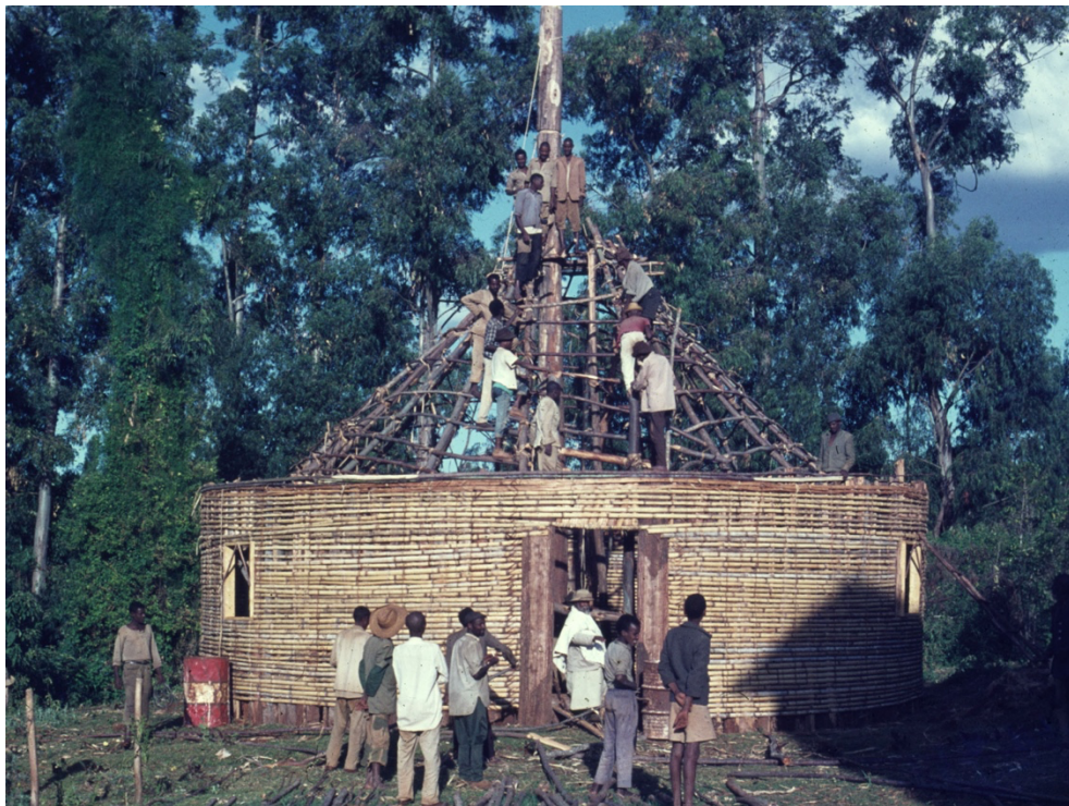
After a brief setback, the centerpost is re-installed.
