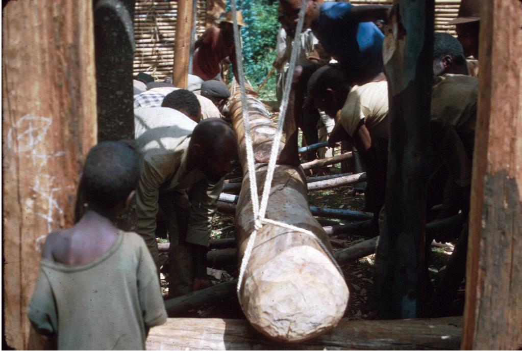
Hauling in the centerpost (wofincha) requires a team of workers.
