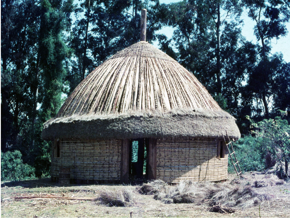
Thatching the roof is a spiral weaving process in which grouped thatch is woven to the roof framing.
