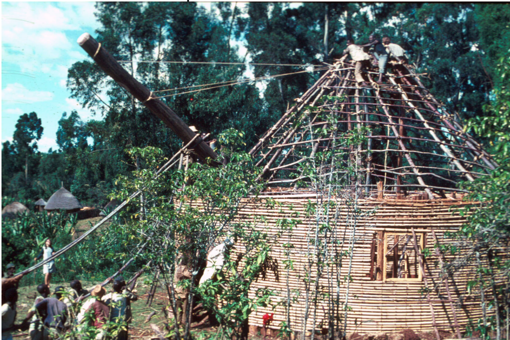
The centerpost is lifted above the walls
