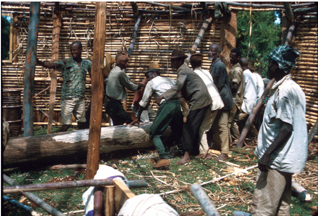
View of workers hauling the centerpost in place.
