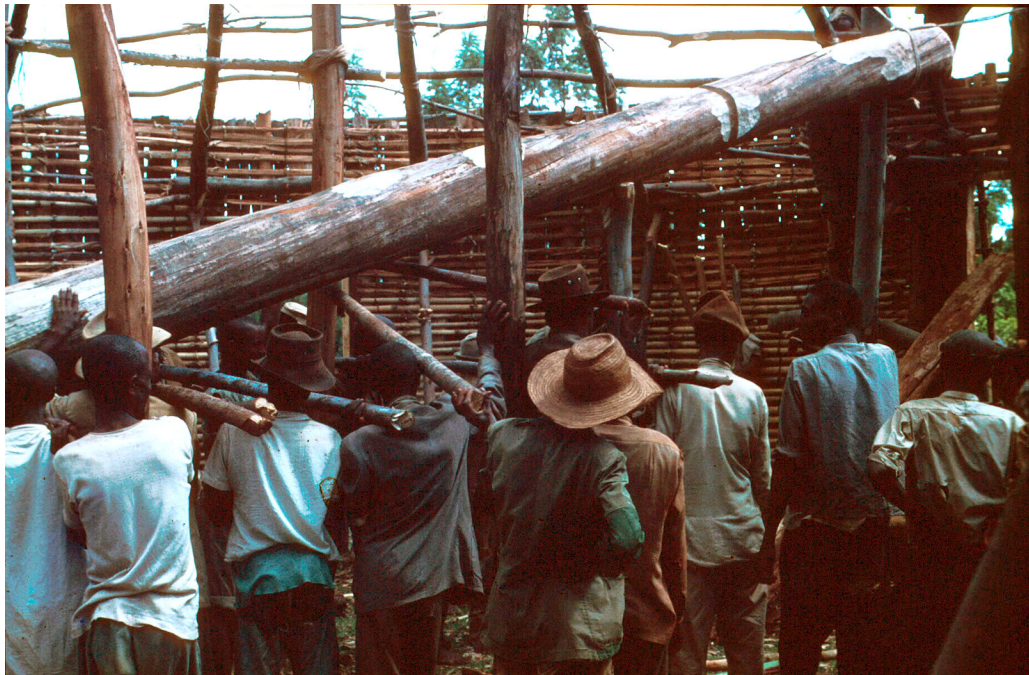
The centerpost is lifted above the circular wall.
