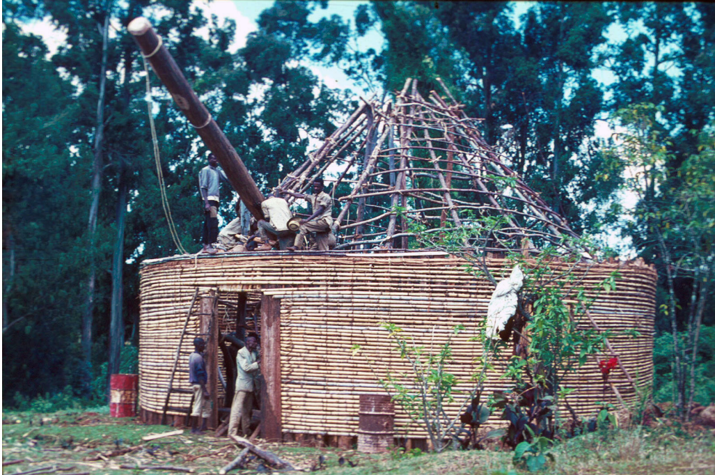
The centerpost is lifted above the walls
