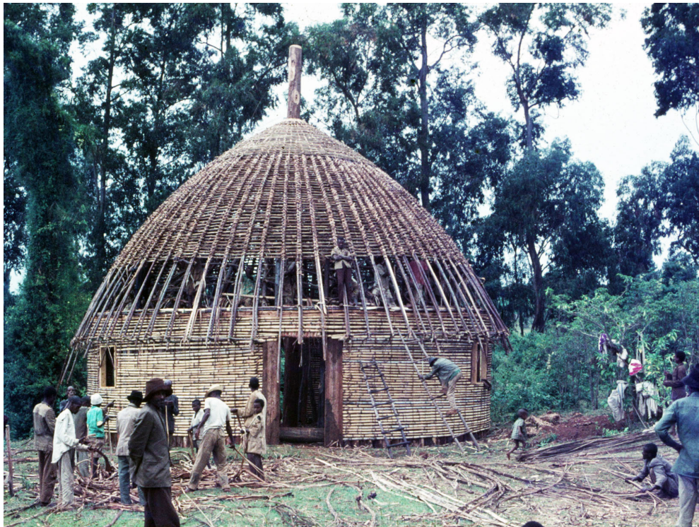
Once the centerpiece is lashed in place, the framing of the thatched roof is undertaken to give a bulbous shape to the roof.
