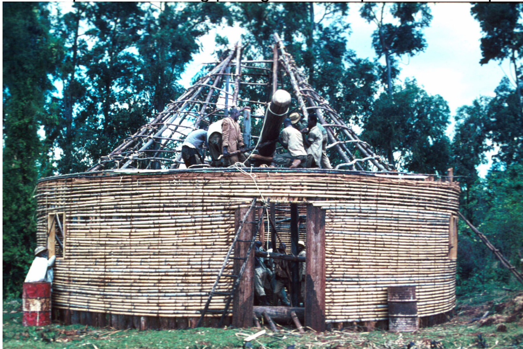
Workers atop the scaffolding pulling the centerpost to vertical position.
